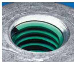
Repaired thread
